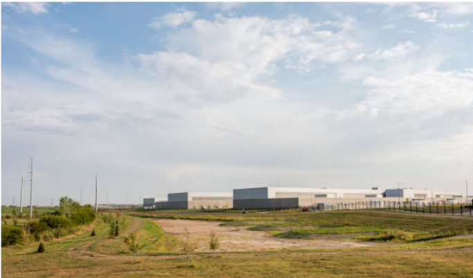
Meta's data center outside Omaha. (Misty Prochaska for The Washington Post)
