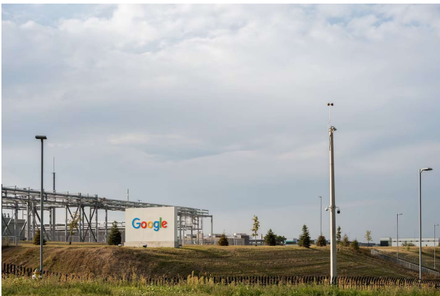
A sign outside the Google data center in Papillion, Neb. (Misty Prochaska for The Washington Post)
