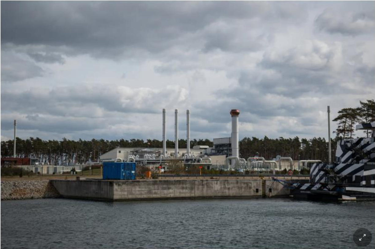
Nord Stream 1 in Lubmin. The pipeline came online in 2011. Germany wanted cheap, reliable energy, and Russia wanted to reduce its reliance on gas pumped west through Ukraine. Lena Mucha for The New York Times
