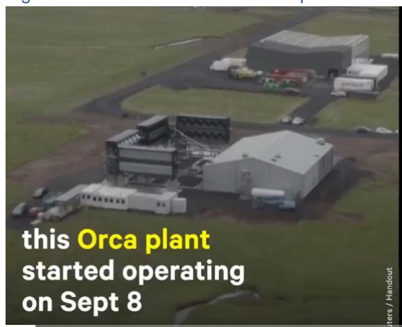
Figure 53: Climeworks Direct Air Capture Plant
