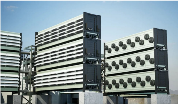
Mammoth's CO 2 collector containers – three of them stacked onto one foundation.
