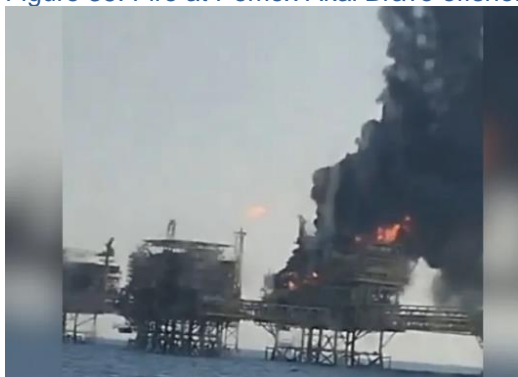
Figure 35: Fire at Pemex Akai Bravo offshore platform in Campeche complex
