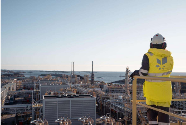
The processing plant at Kollsnes in Øygarden to the west of Bergen Photo: Ole Jørgen Bratland / Equinor
