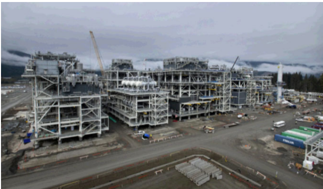
The LNG Canada facility under construction on Sept. 28.
