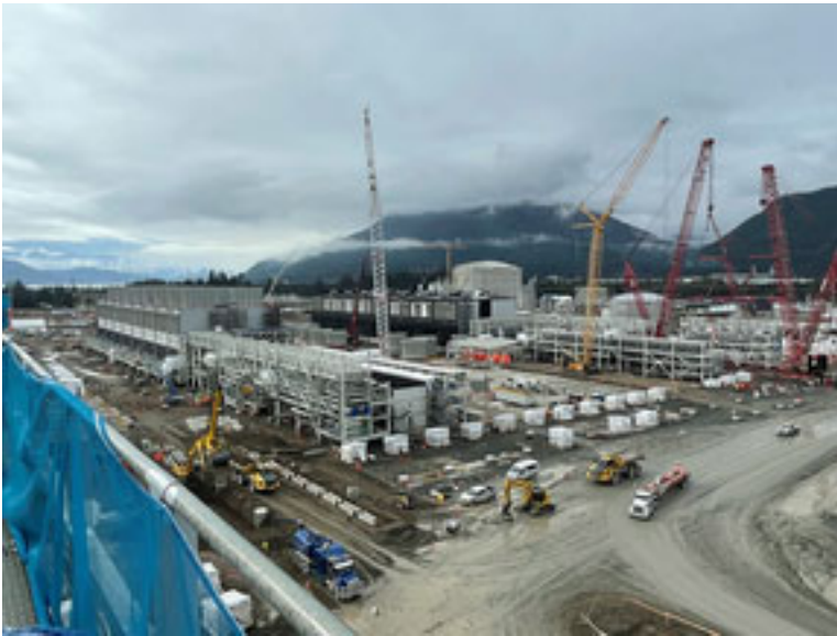
A view of the LNG Canada site. PHOTO BY
