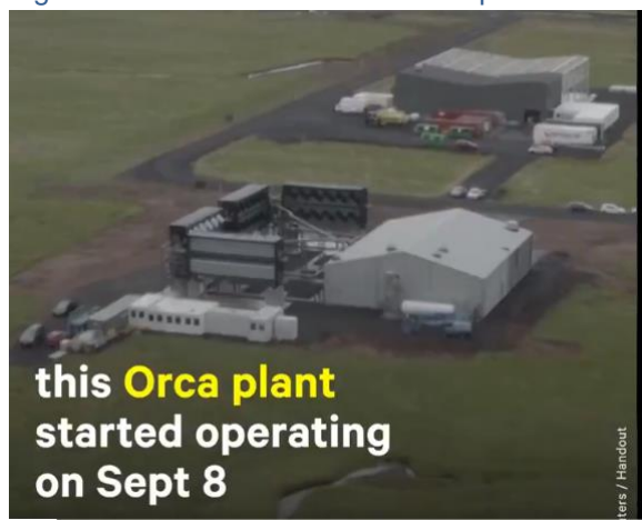
Figure 45: Climeworks Direct Air Capture Plant
