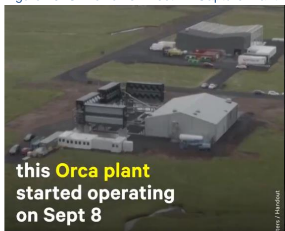
Figure 29: Climeworks Direct Air Capture Plant
