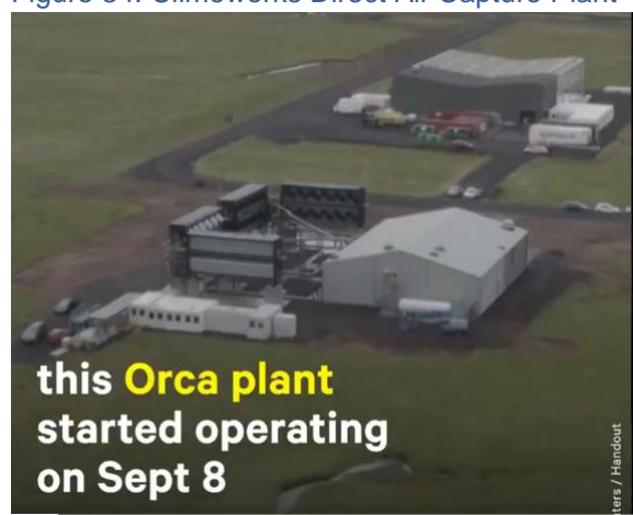
Figure 34: Climeworks Direct Air Capture Plant
