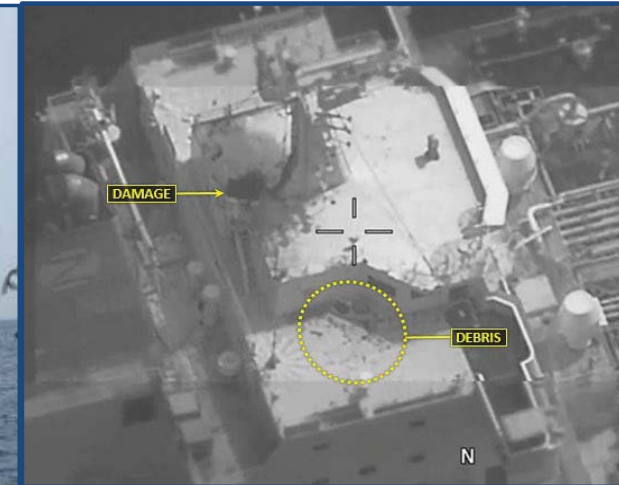
(U) Damage Caused by Iranian UAV Attack
